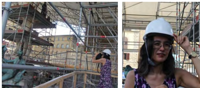
Dr. Else in the scaffolding of Bartolomeo Ammannati's Neptune Fountain (1560-74).
